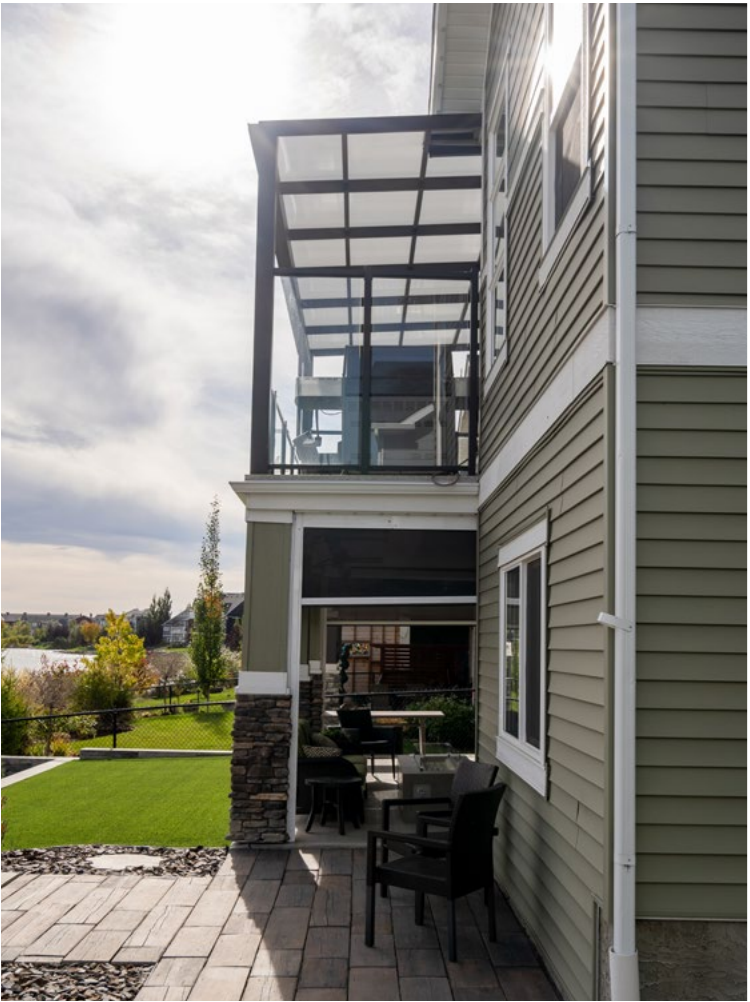
POLYCARBONATE ROOF
